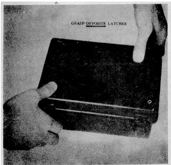
Figure 2-3. Removing KA-3 Keyer Adapter cover.
